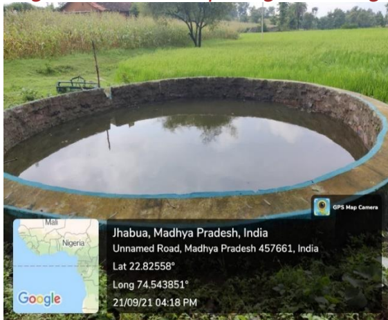
Figure 11: Well deepening and lining
