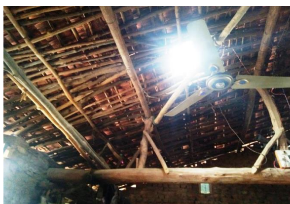
Figure 43: Fiber sheet in beneficiary kitchen
